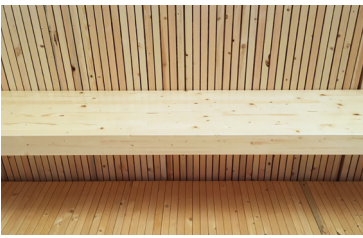
Buildings are crafted with dowel-laminated timber and other eco-friendly products without toxic adhesives or VOCs
